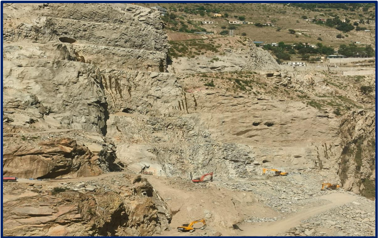
Left Bank Dam Abutment
