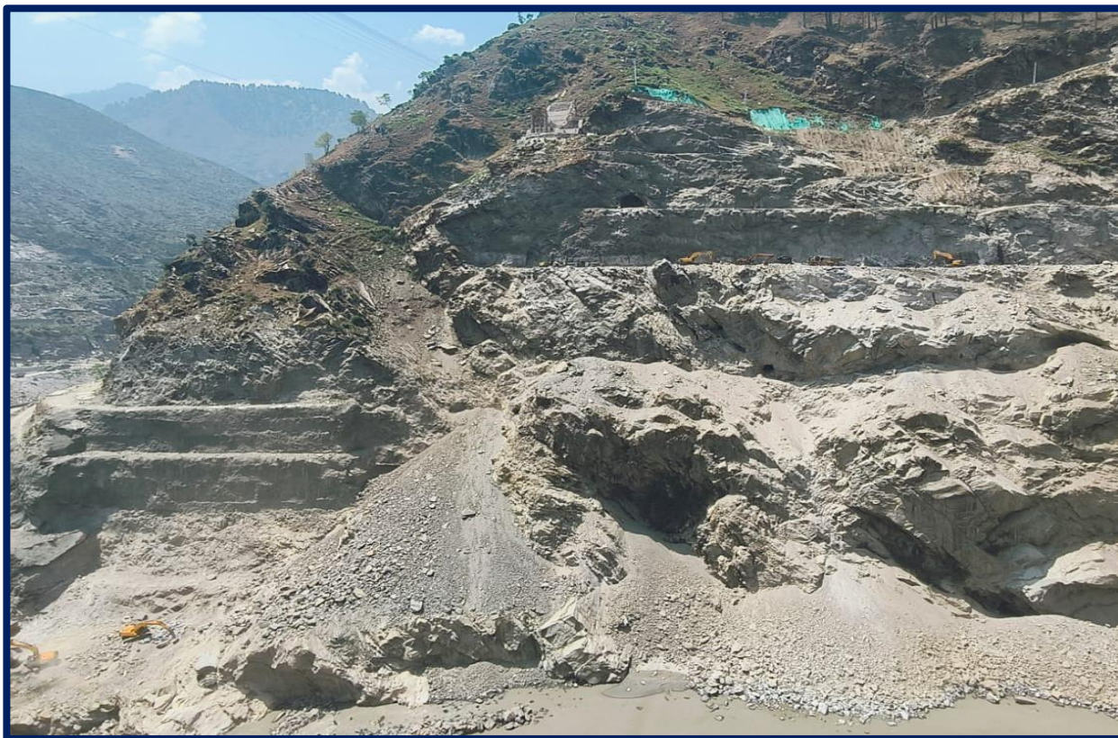
Right Bank Dam Abutment
