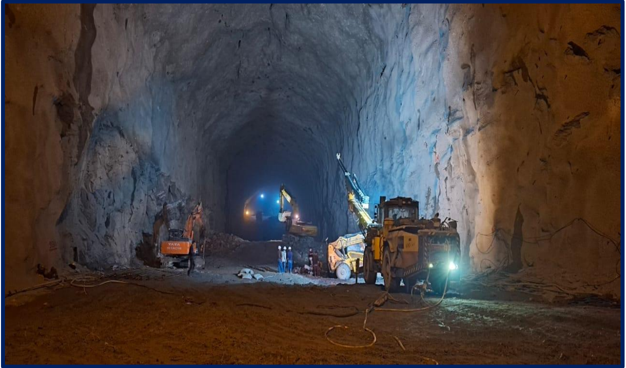
Power House Cavern Excavation
