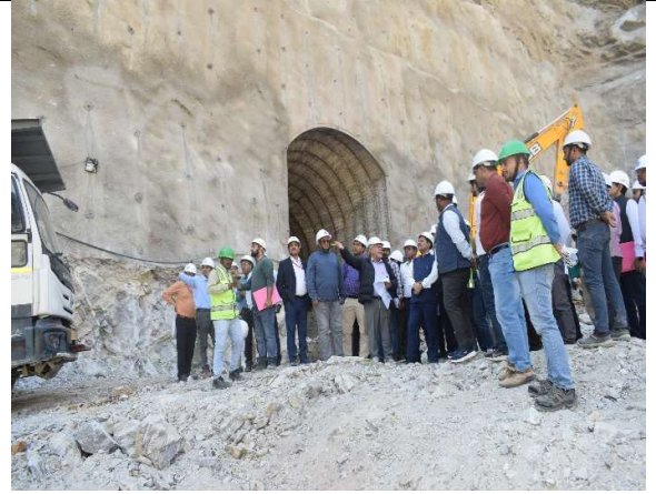
Inspection of Power Intake
